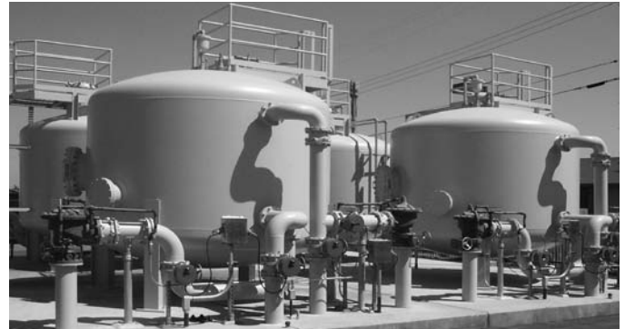
MetalEase-61 Installation in Elk Grove, California
